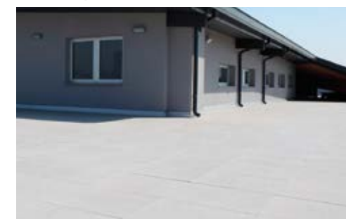
Posa sopraelevata . Raised installation
